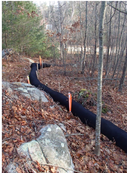
Erosion control protecting wetland
