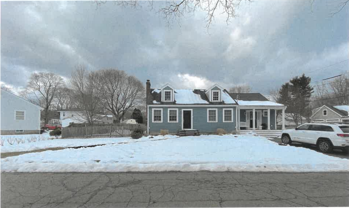
FRONT FAÇADE (EAST)
