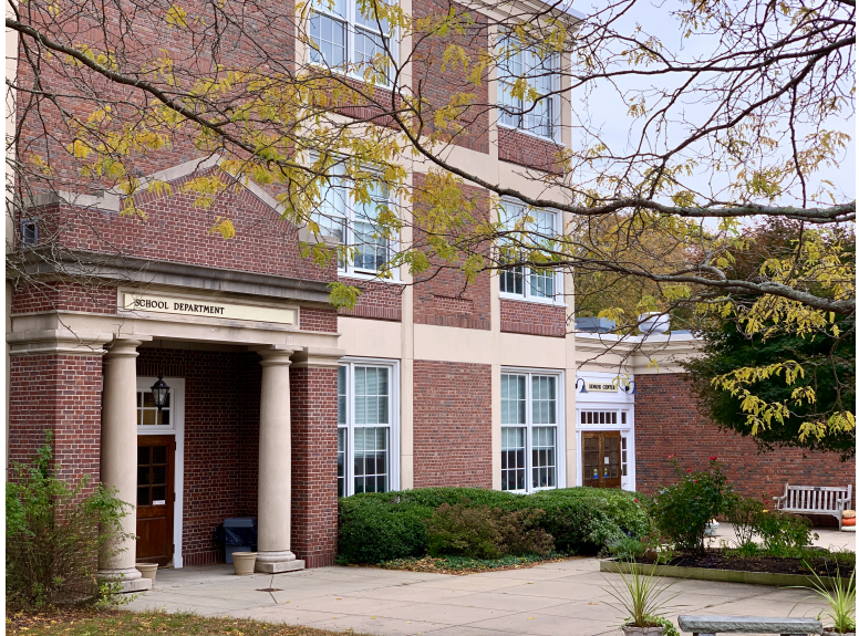
and will eventually need renovation/addition(s) training Hingham School Department Offices
