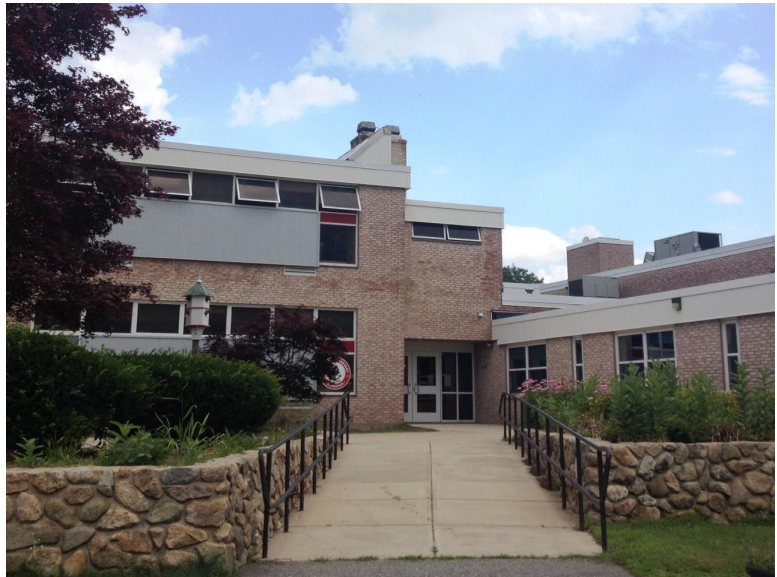
The Foster School has been identified as one of the municipal buildings most vulnerable to flooding from sea level rise. Plans are underway to rebuild it away from the flood zone area.
